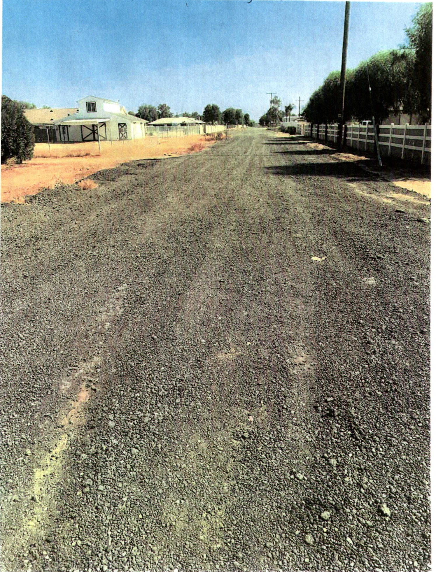
DOWSON RD @ ELLIS AVE LOOKING SOUTH.
