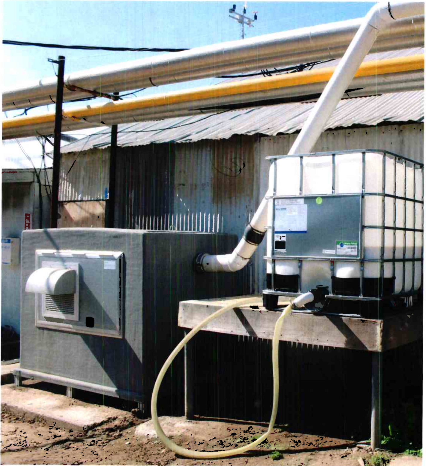
Autumn Brands uses vapor phase technology to neutralize cannabis odors before they leave the property. Photo by Kathryn Barnes/KCRW.
