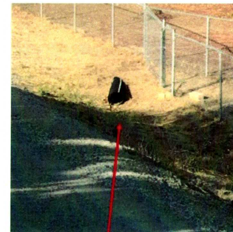
Applicant's non-permitted drainage system encroachment in part of Cibola Circle
