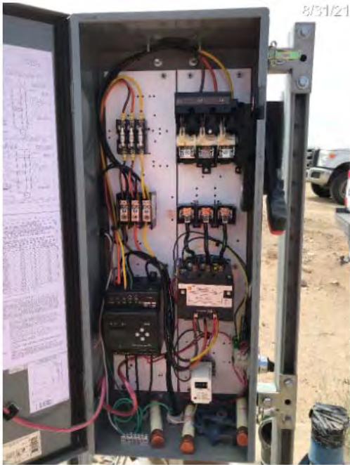
E1 Salvage Existing Electrical Control Panel Not To Scale
