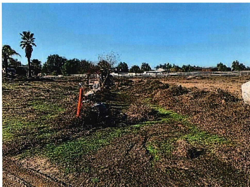
Photo 8: Looking southwest (downstream) at swale within the property. This section has manmade bed and bank and has rocks placed on the top of the bank.
