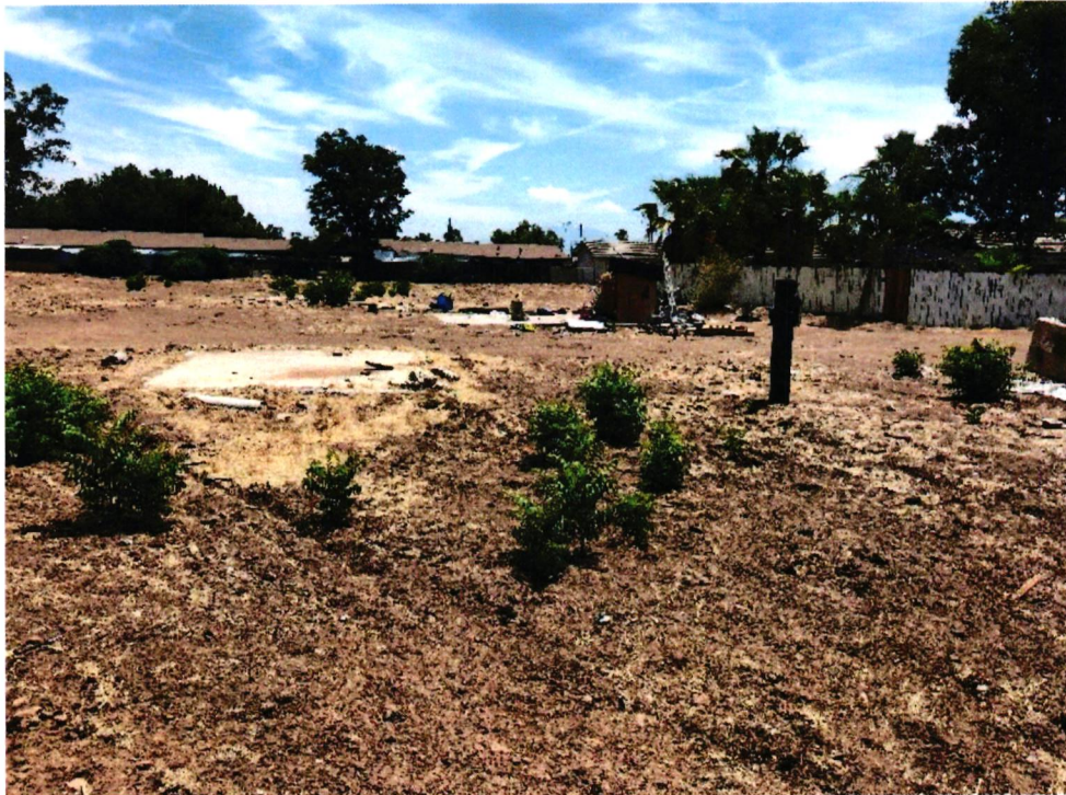
Figure 6. Poured foundation remnants. (facing)
