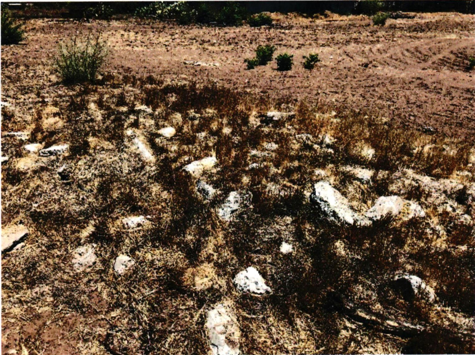
Figure 7. Debris pile of concrete chunks (facing View from NW corner.)
