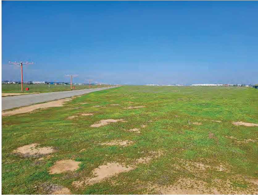
11. View of adjoining MARB flightline and runway, from south facing north
