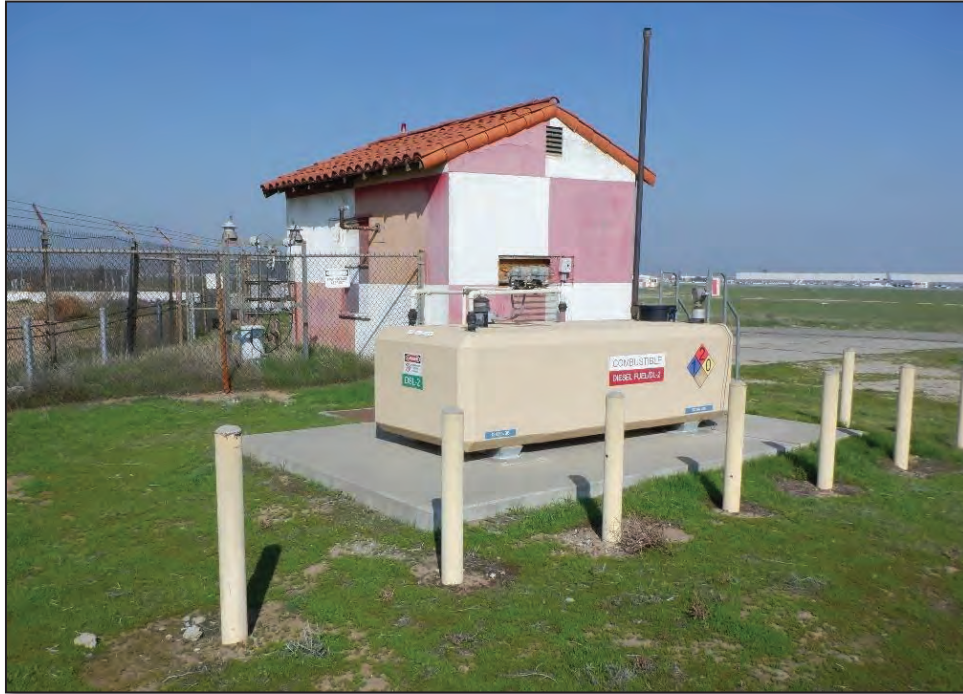
Photo 6 West and south elevations of Utility Building #1300 (facing north)
