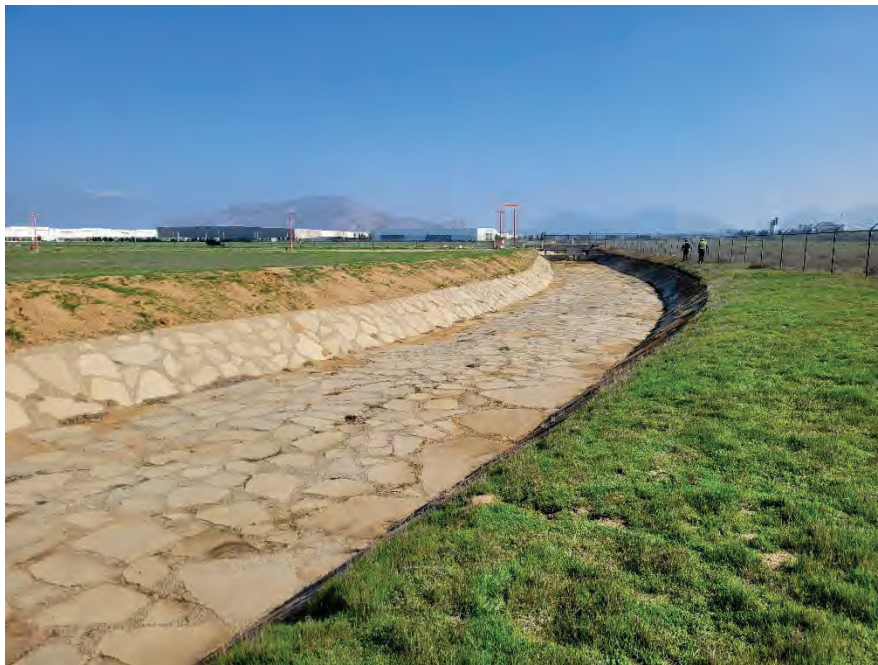
10. View of paved streambed in southern portion of Site
