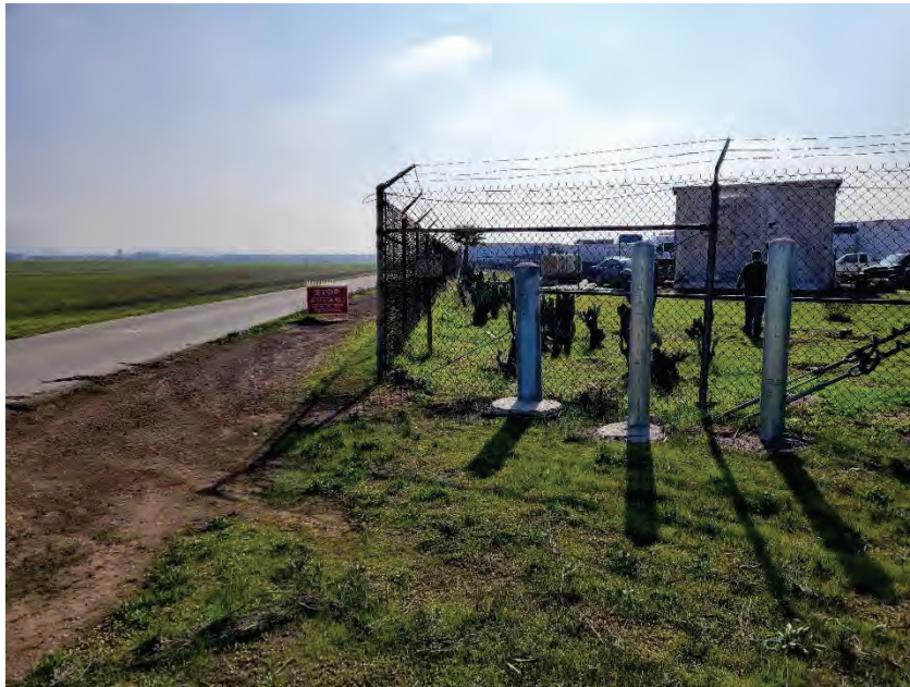
7. View of high-pressure gas pipeline signage at 5137 Patterson Avenue
