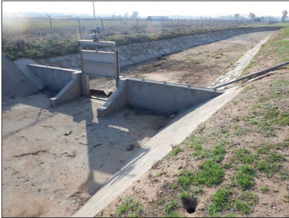
Photo 4 Overview of P-33-024867 (facing southwest)
