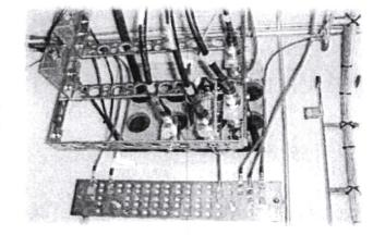
below shall be effectively bonded back to the internal grounding (earthing) system with a 16 mm<sup>2</sup> csa (#6 AWG) or coarser equipment grounding conductor by using the following requirements and connection methods described within this document:
