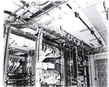
equipment and help maintain adequate separation between the cable groups. The orderly separation and support of cable also simplifies maintenance. All cables installed in cable trays shall installed in a neatly secure
