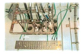
below shall be effectively bonded back to the internal grounding (earthing) system with a 16 mm2 csa (#6 AWG) or coarser equipment grounding conductor by using the following requirements and connection methods described within this document:
