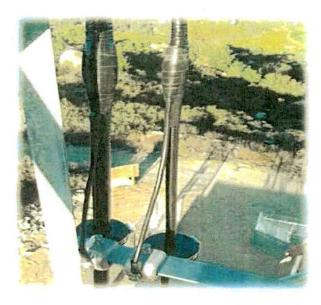
section 1.4). This will require the installation of a grounding kit similar to Andrew Type 204989-2 Strap Kit (for Andrew LDF5-50A) or appropriate kit number for the antenna feed line being used. All transmission lines shall be installed and bonded to the tower using ground kits as follows:
