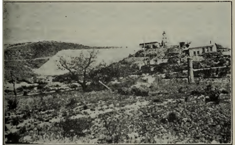
No. 1 Shaft, Temescal Tin Mine, American Tin Corporation, Riverside County.
