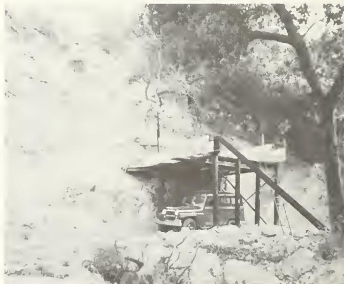
FIGURE 10. Loading chute-bunker at Grapevine clay shale deposit. Loosened clay shale is pushed into bunker from quarry above (figure 9) by bulldozer. This illustrates the typical method used for many years to load trucks at most of the clay deposits in the Corona area. Skiploaders (fig. 18) have replaced this method in most operations. Observer faces southwest.
