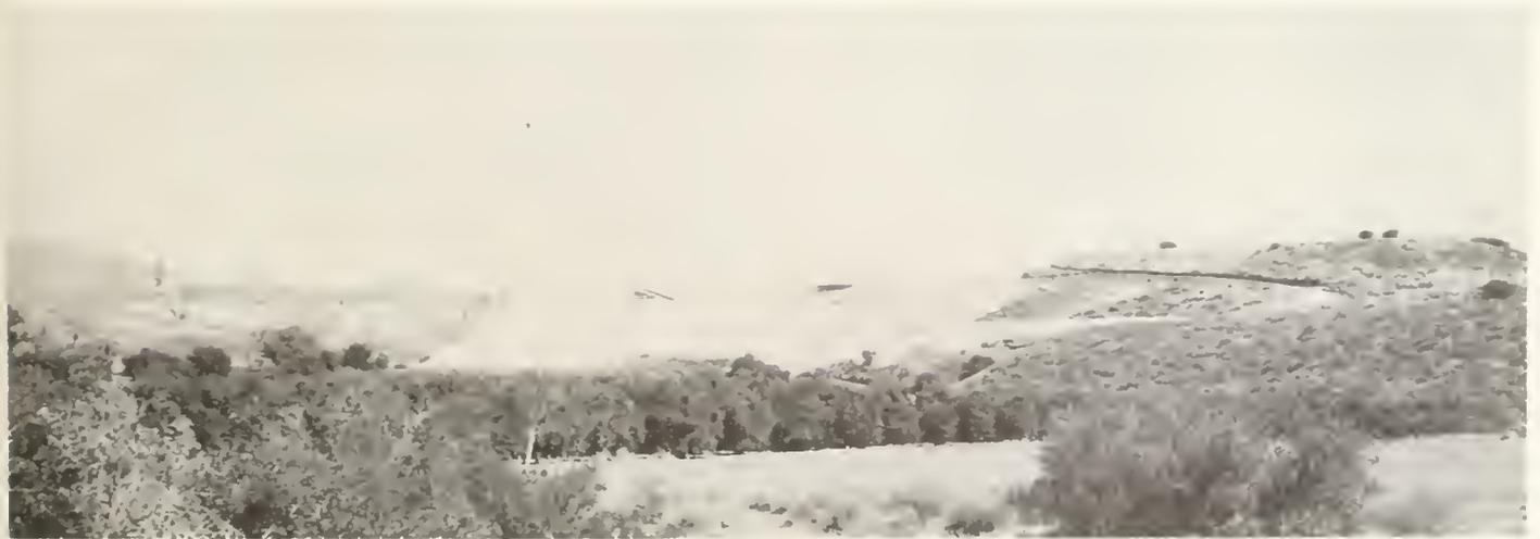
FIGURE 39. Owens-Illinois Glass Company's glass sand operation in the Corona-Elsinore trough, southeast of Corona. Inactive original pit east of highway is at left, present (1958) active pit at center and top of plant barely visible beyond. Pits are opened in Paleocene Silverado formation sandstone which is overlain by a thin covering of terrace deposits on the flat-topped ridges at both left and right. Observer faces southeast.
