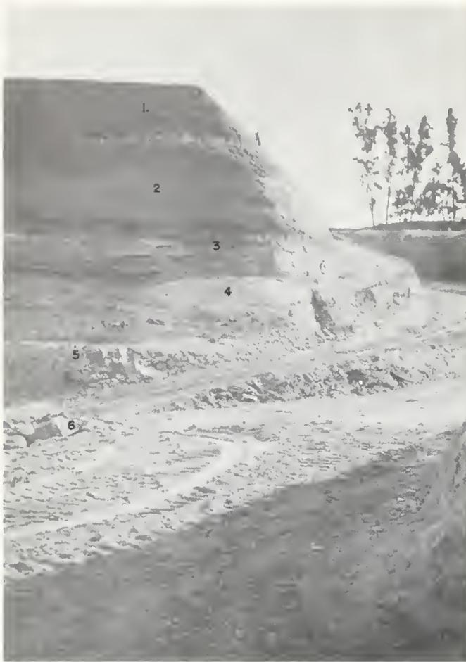
FIGURE 15. Exposure of Silverado formation sandstone and clay at the Bedford Canyon clay mine of Gladding, McBean and Company. Hornblende diorite (6), a phase of the Corona hornblende diorite porphyry, is overlain by residual red mottled clay (5), arkosic sandstone (4), sedimentary red mottled clay (3), coarse arkosic sandstone (2), and sandy older alluvium (1). Observer faces southwest. *Photograph by George B. Cleveland.*
