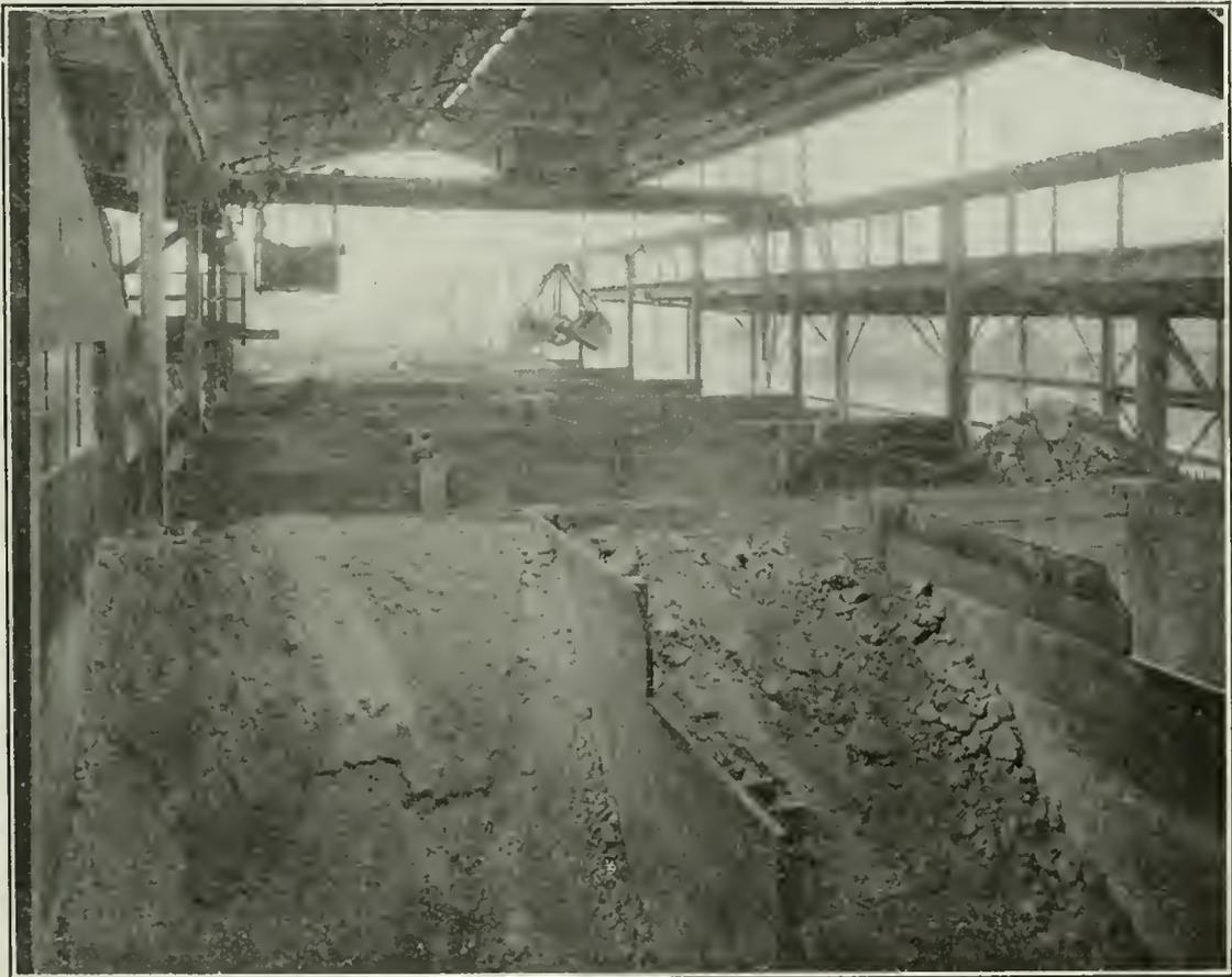
PHOTO No. 20. Clay bins and unloading crane, Lincoln Heights plant, Pacific Clay Products Co., Los Angeles. (Photo by courtesy of the company.)
