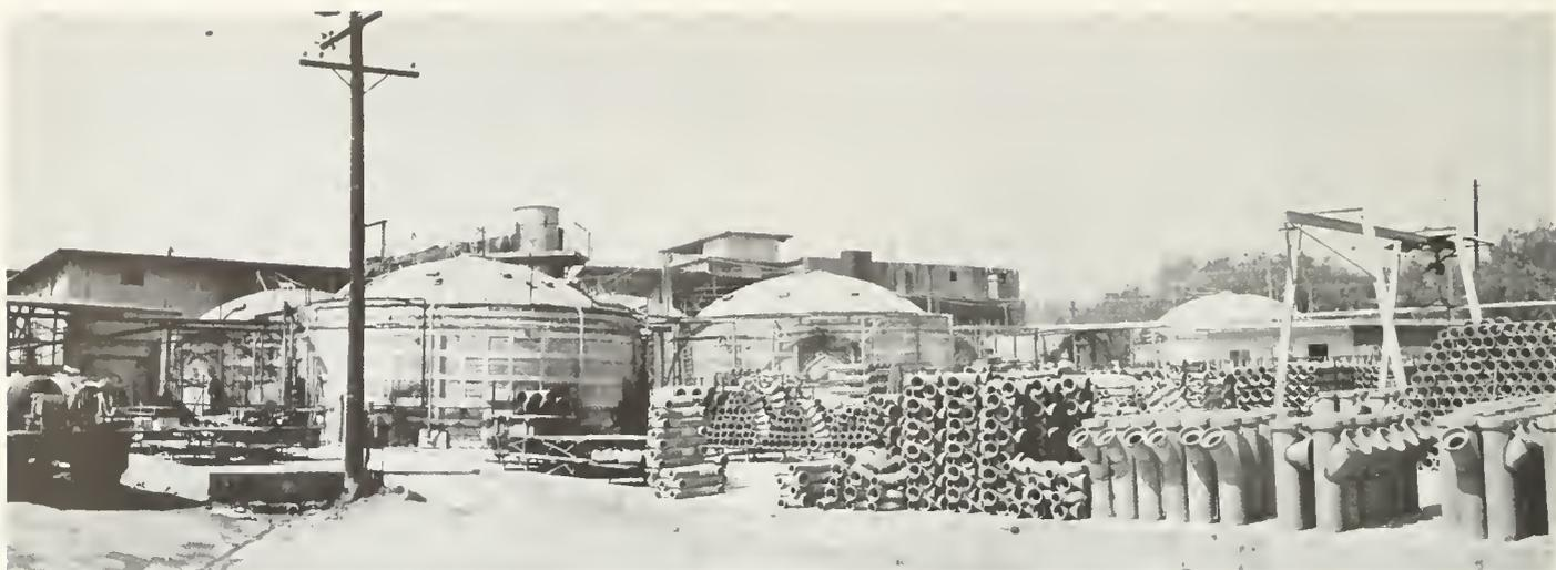
FIGURE 21. Clay pipe manufacturing plant of Tillotson Refractories Company, Corona. Raw material is ground, pugged and extruded to form clay pipe in building in background. Also in this building the pipe is glazed and dried by gas heat. The pipe then goes to periodic "beehive" kilns (center) for firing. Finished pipe is stored in yard (right foreground) to await truck shipment to users. Observer faces southwest.
