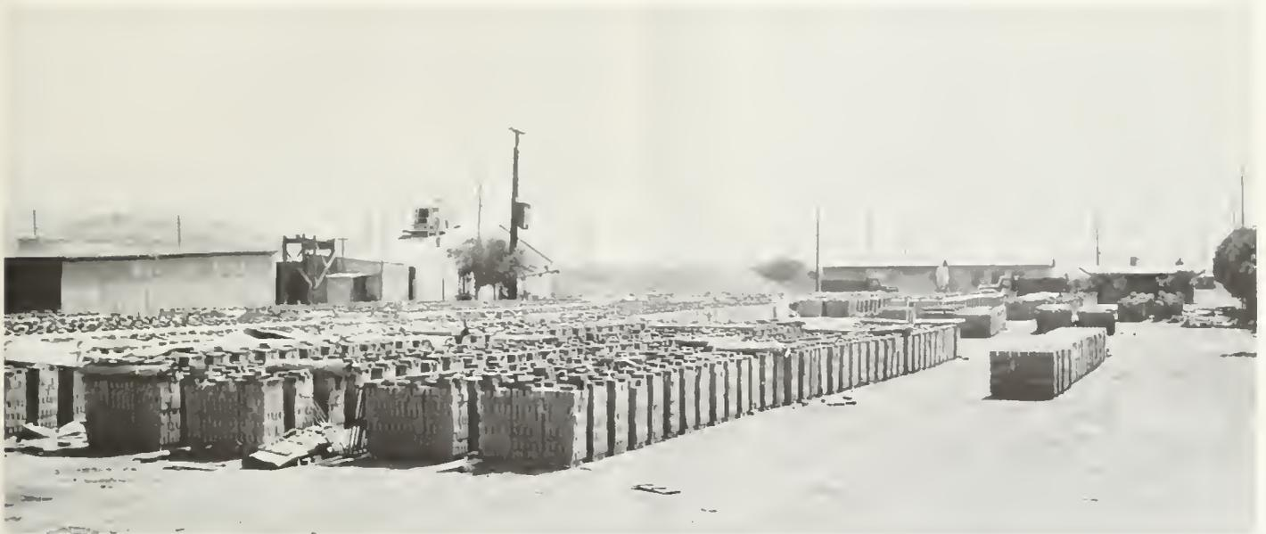
FIGURE 13. Plant and finished brick storage yard of Liston Brick Company, lower Bedford Wash. Plant (left background), raw clay stockpile (center background), office and shop (right background), finished brick storage in foreground. Observer faces southwest.
