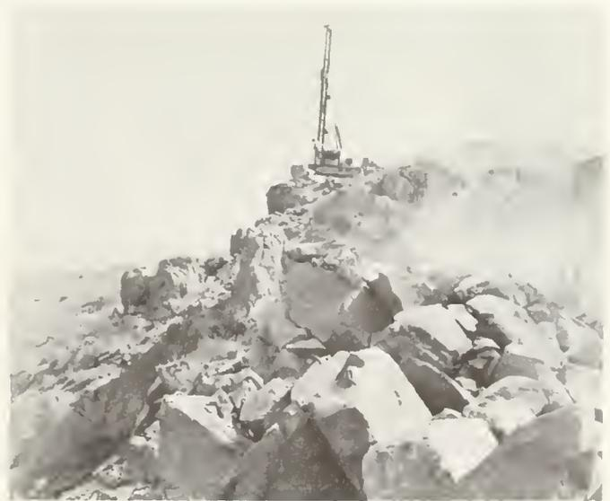
FIGURE 28. Blast hole drilling with Joy rotary-air-blast drill (top center) and secondary breaking with jackhammer (middle right) at Temescal Canyon rock quarry, north pit. Observer faces northeast.
