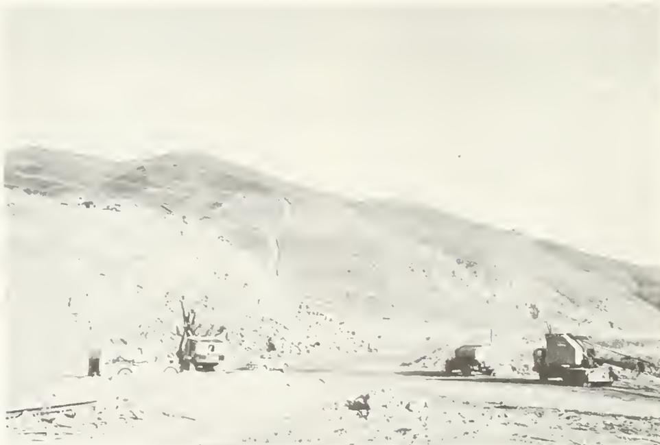
FIGURE 26. Temescal Canyon rock quarry of Matich and Sundt Company, eastside of Temescal Wash. Granodiorite (Corona hornblende granodiorite porphyry) of Jurassic or Cretaceous age was obtained from north quarry (left foreground) and south quarry (right middle ground) during 1957, for use in facing a levee along the Santa Ana River west of Riverside. Jurassic quartz latite (Temescal Wash quartz latite porphyry) was also obtained from the south quarry. Observer faces southeast.
