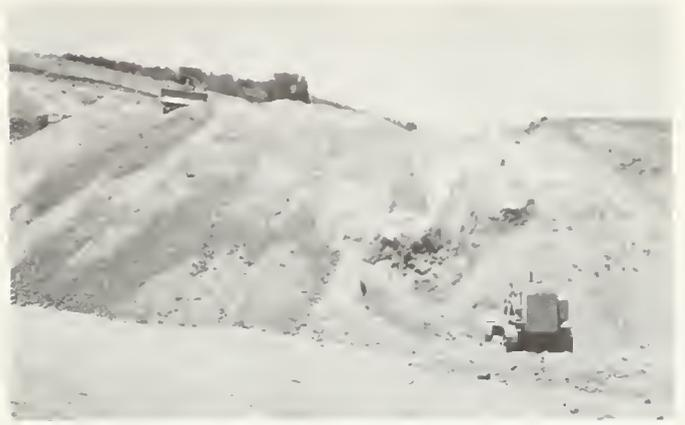
FIGURE 17. Clay shale stockpile, Sky Ranch Clay Company mine, west pit. Ripper-bulldozer (upper left) loosens the clay shale and pushes the loosened material to the stockpile from which a skiploader (lower right) loads trucks. Observer faces north.
