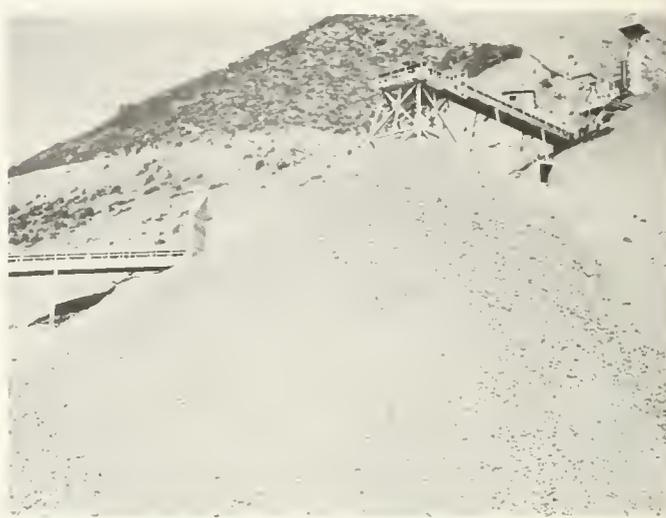
FIGURE 34. Raw material surge pile, Minnesota Mining and Manufacturing Company, Temescal Canyon. Quartz latite porphyry is delivered to the surge pile (center) by belt conveyor from the primary crusher (upper right) at quarry floor level. Belt conveyor (left) moves the crushed rock from the surge pile to the plant (fig. 31) below. Observer faces northeast. *Photograph courtesy of Minnesota Mining and Manufacturing Company, St. Paul, Minnesota.*
