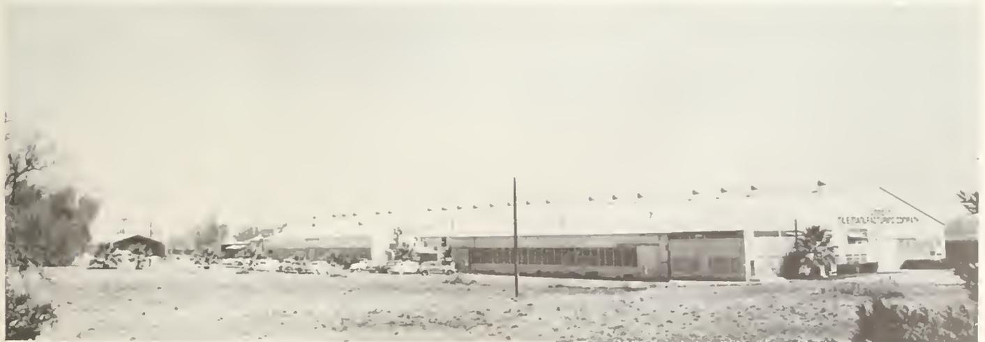
FIGURE 11. Jordan Tile Manufacturing Company plant, Corona. Raw material storage is in open building at left background. Large building houses pugging machines, presses, tunnel kilns, storage and shipping facilities and offices. One of the first clay pipe manufacturing plants in the Corona area—the Pacific Clay Manufacturing Co. (fig. 1)—occupied this site from about 1900 to early 1920's. Observer faces northwest.
