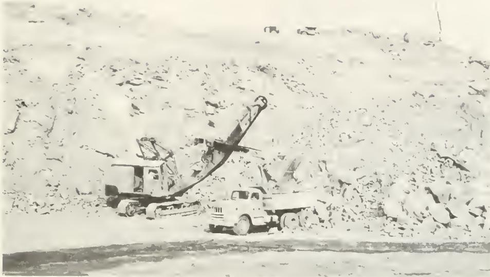
FIGURE 27. Loading blasted-down rock at north pit of Matieh and Sundt Company's Temescal Canyon rock quarry. Vertical blast holes are drilled from above (rock drill and compressor, upper right). Six-wheel dump trucks transport the material to job site or to stockpile area in Temescal Wash where the rock is sized by means of bulldozers and secondary breaking is done with drop balls operated from truck-mounted cranes. Observer faces east.
