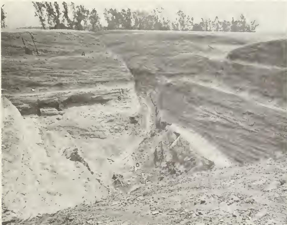
FIGURE 7. Bedford Canyon clay mine of Gladding, McBean and Company, during initial development in early 1955. Hornblende diorite (D) is overlain by residual red mottled clay (C, mapped with the Paleocene Silverado formation), Silverado formation arkosic sandstone (S), and older alluvium (A). Observer faces southeast. Photograph by David P. Shelhamer, Los Angeles, California, courtesy of Gladding, McBean and Company, Los Angeles, California.
