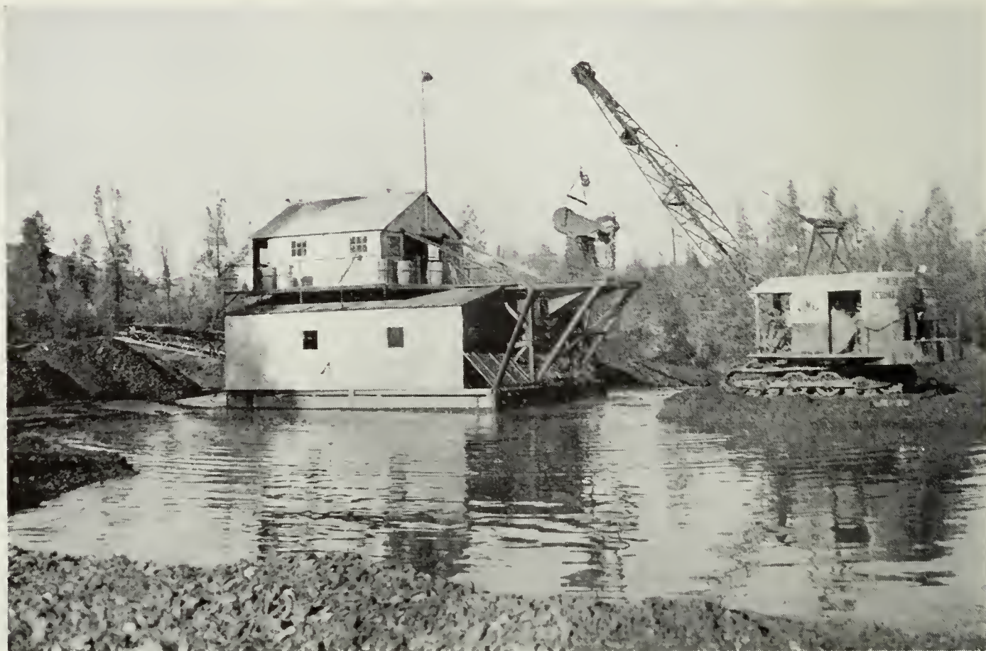
PHOTOGRAPH 11. Dragline dredge of Pioneer Dredging Co.
