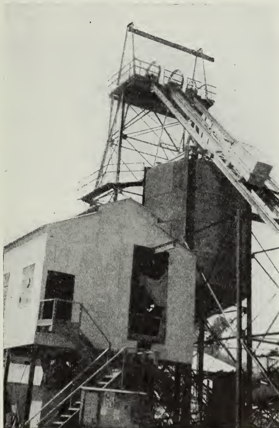
Steel headframe at Big Canyon Mine of Mountain Copper Co.
