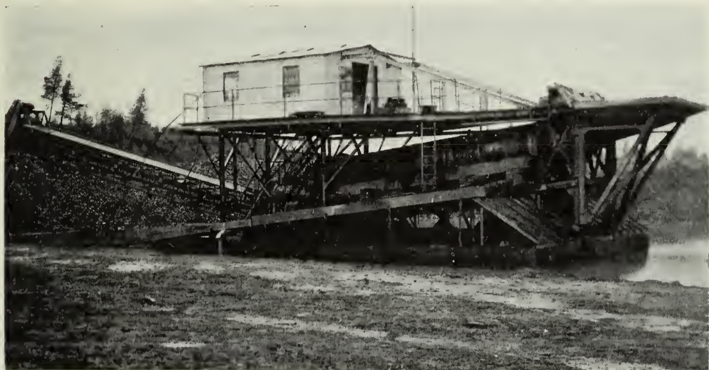
PHOTOGRAPH 8. Carlson and Sandburg dragline dredge for 3-cubic yard shovel. (Photo by courtesy Bodinson Mfg. Co.)
