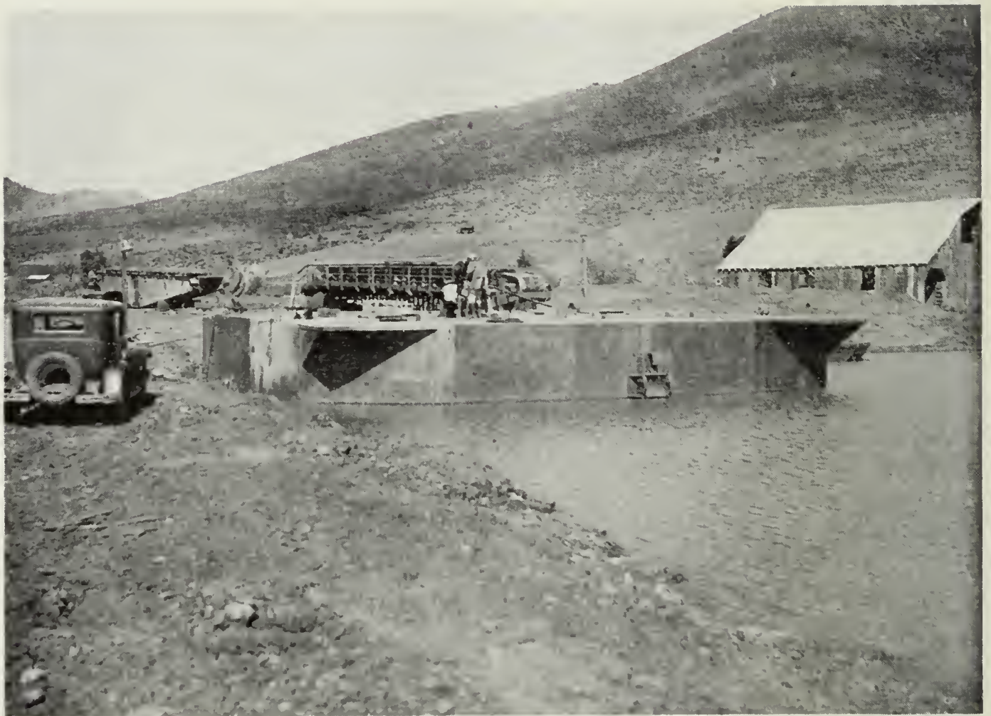
PHOTOGRAPH 13. Steel hull of dredge of Yreka Gold Dredging Co.
