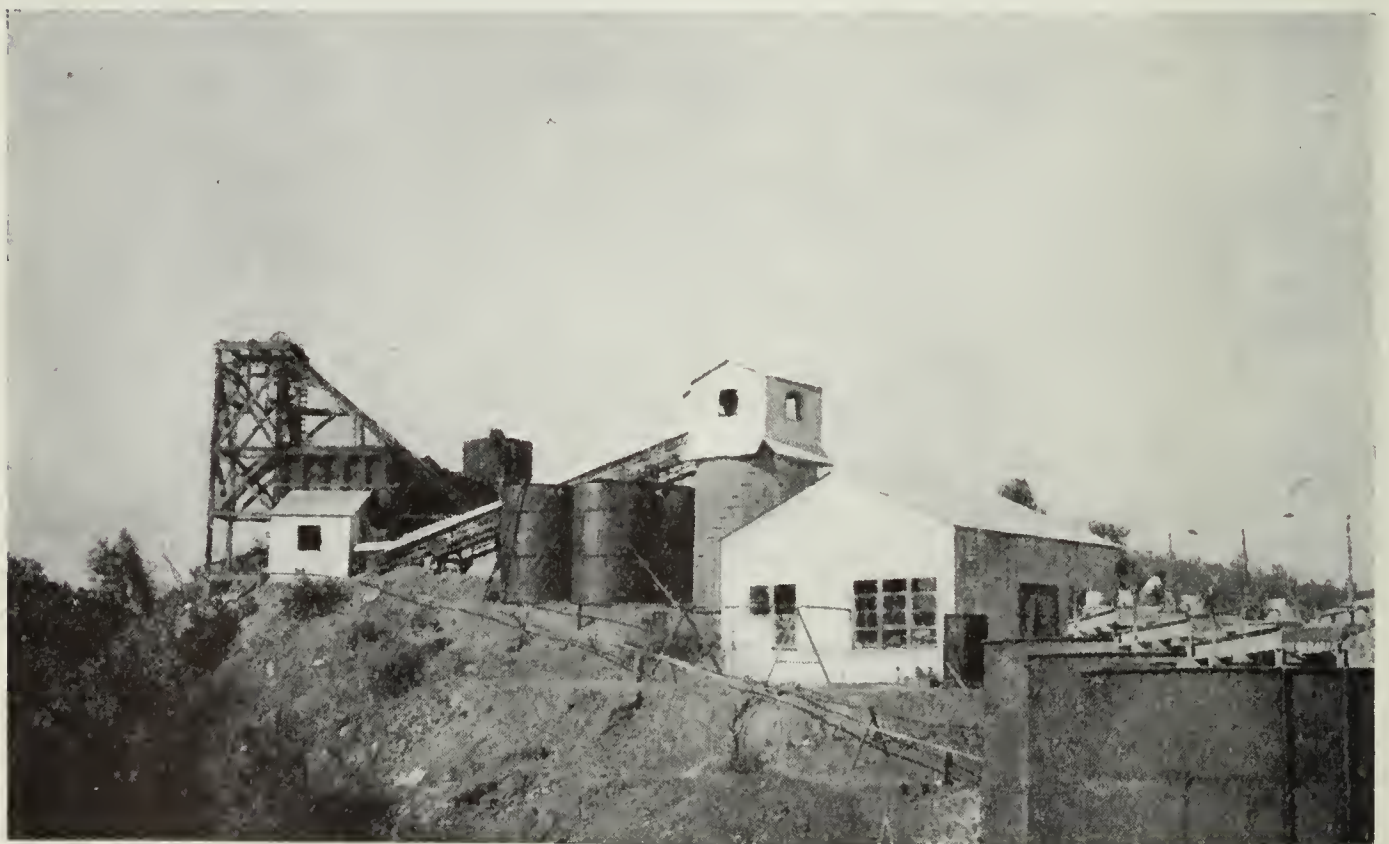
Surface plant at Crystal Mine, south of Shingle Springs. Steel cyanide tanks in right foreground.
