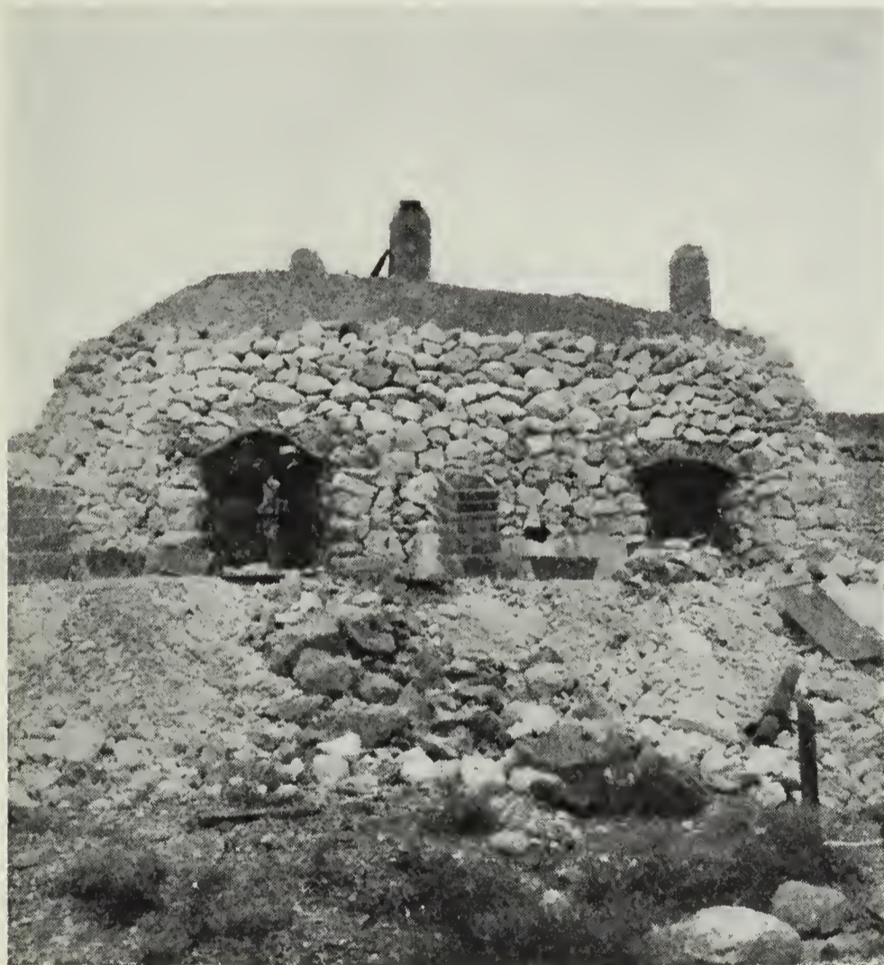
PHOTO. 19. 3-Compartment Sulphur Ovens, Fraction Sulphur Mine, Italo Sulphur Industries Co., Last Chance Range of Mountains, Inyo County.
