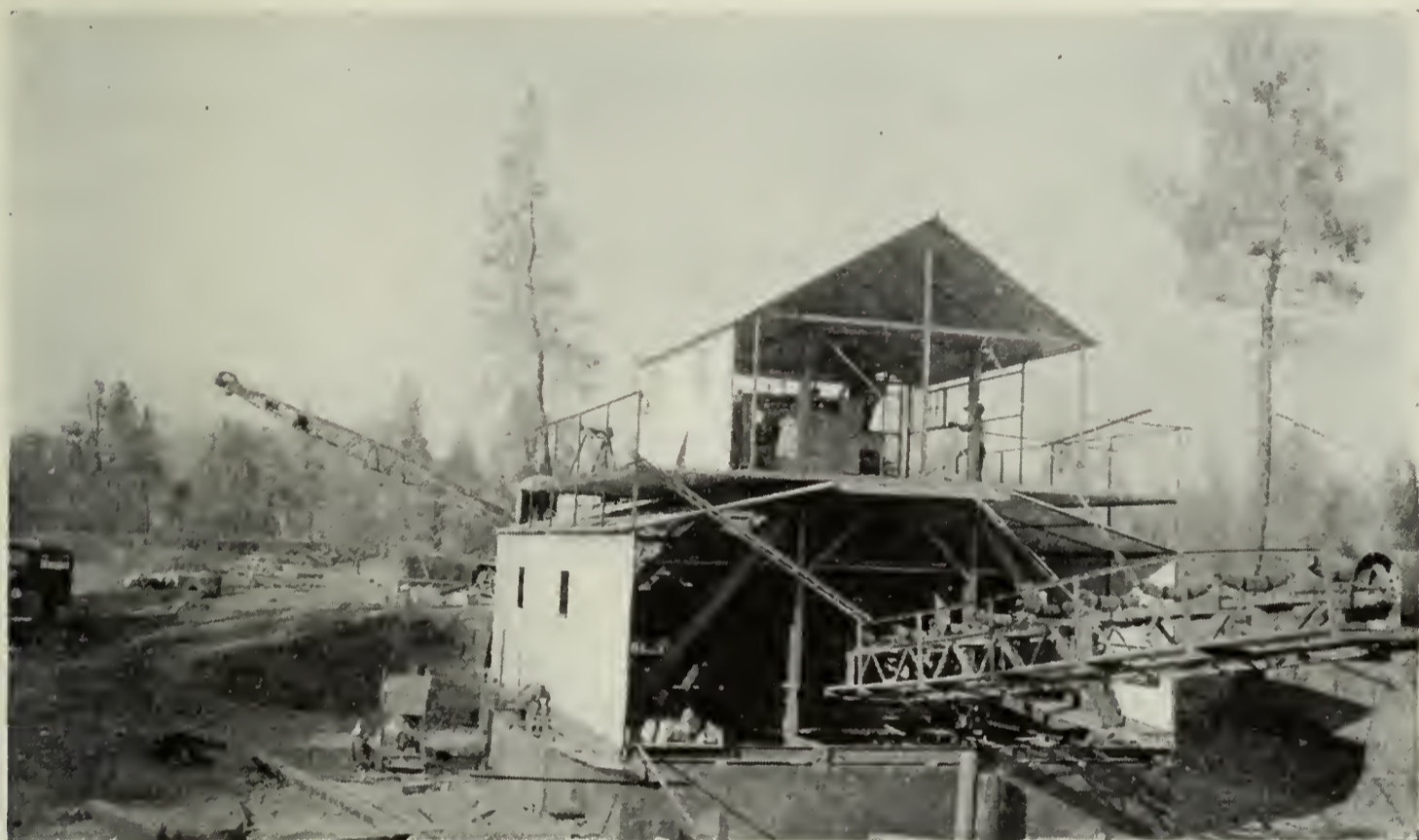
PHOTOGRAPH 6. Dragline dredge under construction in field.
