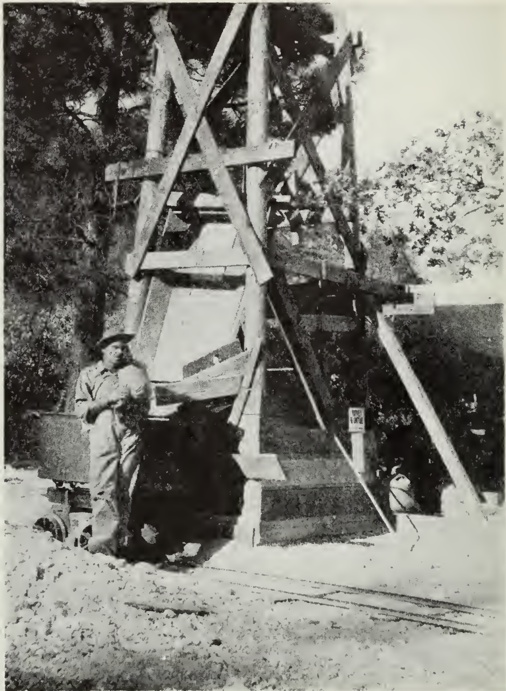
Headframe used in prospecting a shallow gravel deposit at Hinds Mine, Pleasant Valley.
