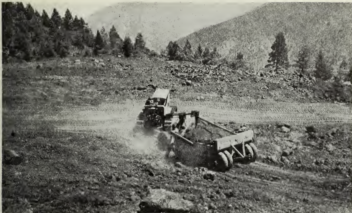
PHOTOGRAPH 3. Carryall and tractor working on top bench of gossan quarry.
