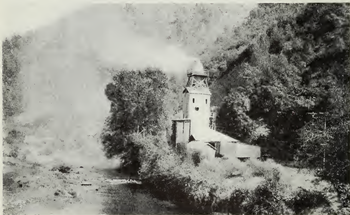
Plant of Pacific Minerals Co., Limited, at Chili Bar on South Fork of American River. Roofing granules are made here from Mariposa slate taken from a deposit adjoining the plant.
