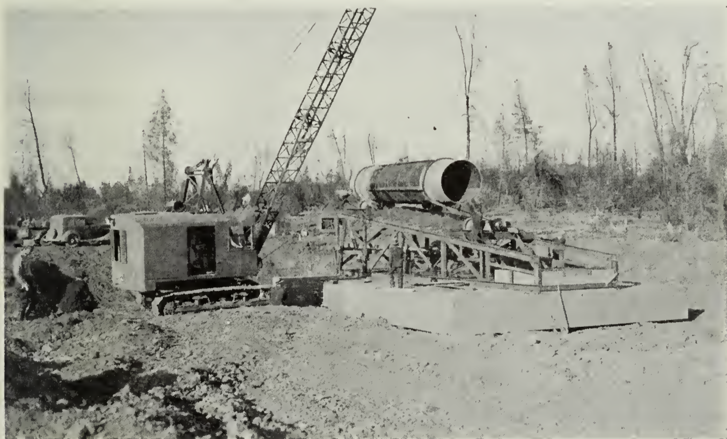
PHOTOGRAPH 7. A. C. Mining Co. dredge under construction.
