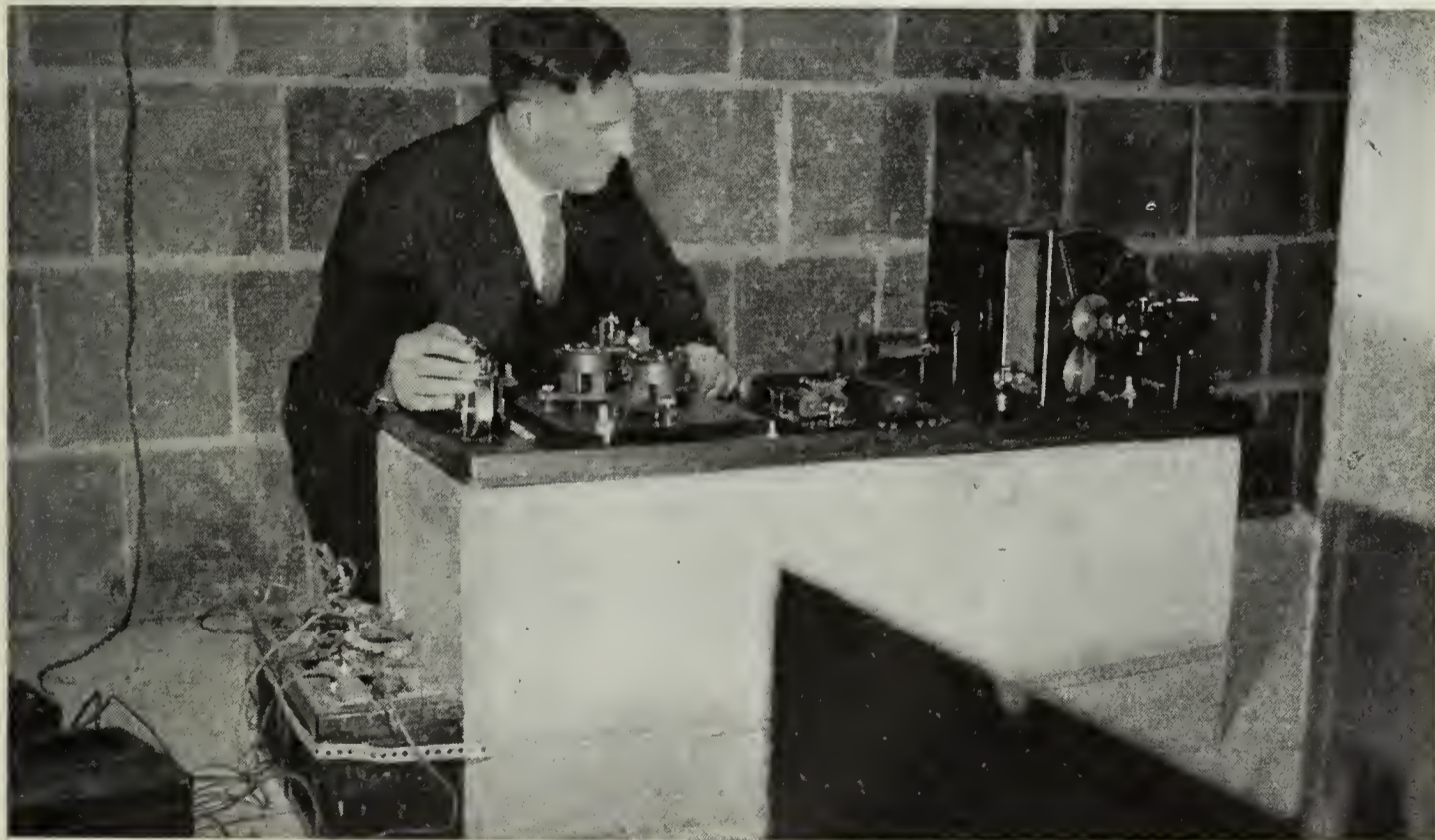
FIG. 5. A strong motion seismograph being installed.
