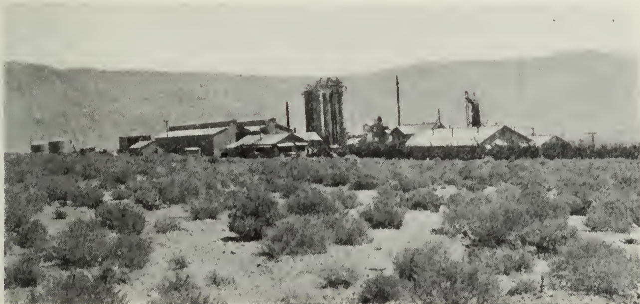
PHOTO. 20. Pacific Alkali Company's Soda Plant, Owens Lake, Inyo County.
