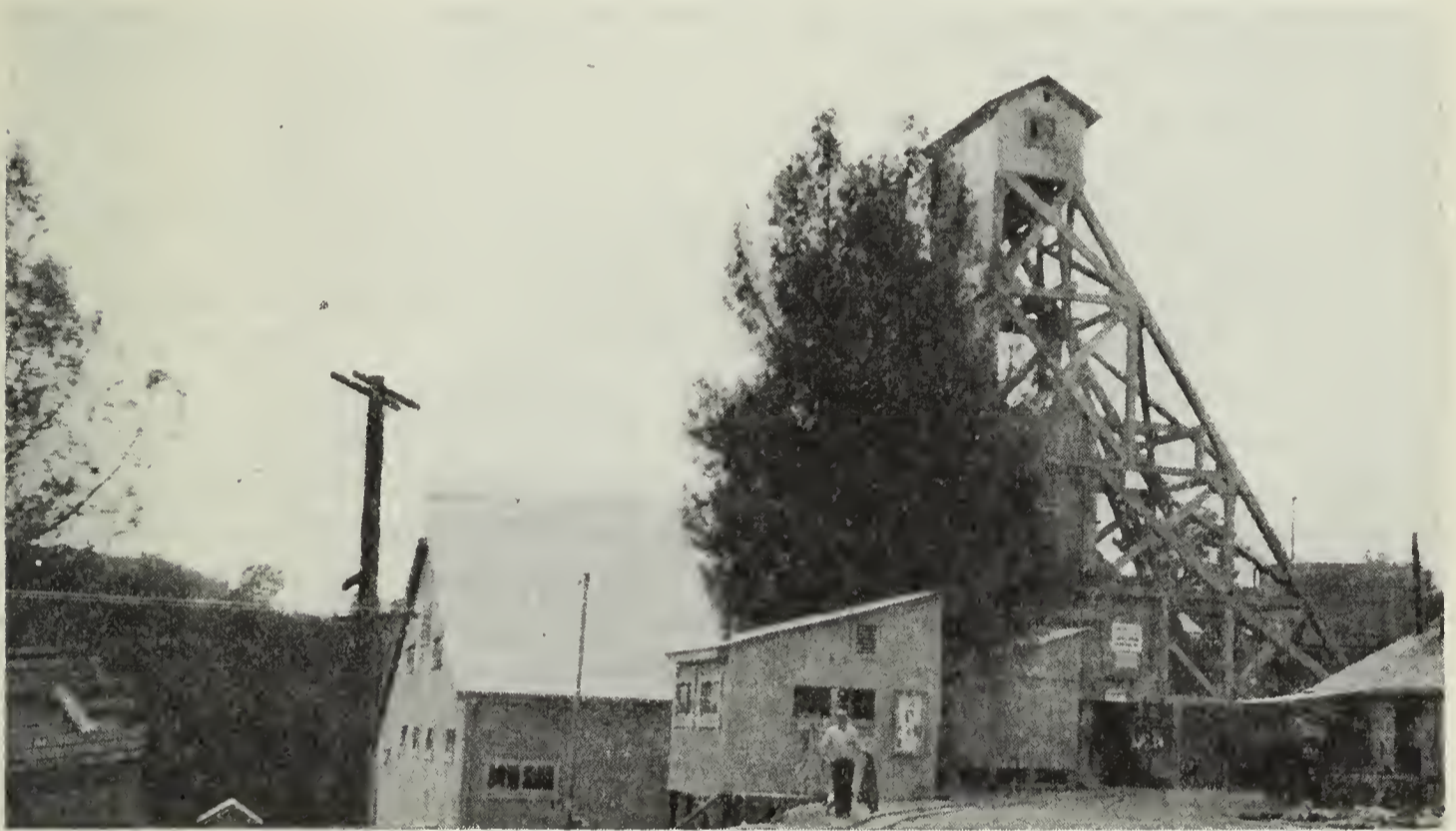
Headframe and mill building at Pyramid (Gold Reserve) Mine, north of Shingle Springs.
