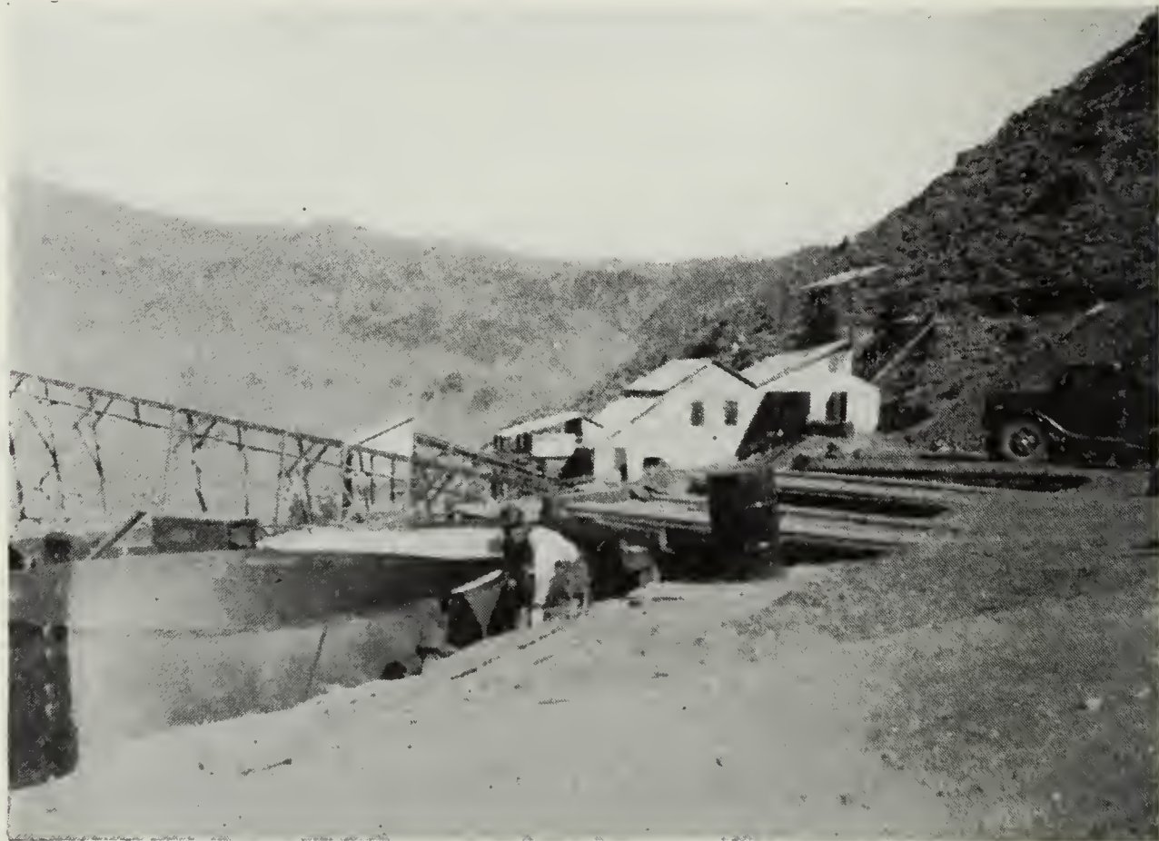
PHOTO. 7. Crushing Plant—Capacity 70 tons. Ruth Mine, Argus Range of Mountains, Inyo County.
