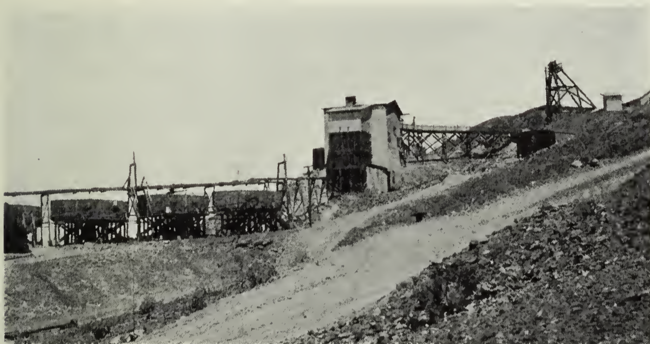
PHOTO. 4. Keeler Gold Mine and Cyanide Plant, Keeler Gold Mining Co., Keeler, Inyo County.
