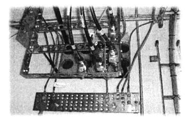
RF transmission SPDs **shall** be bonded to the MGB within 610 mm (24 in.) of entry into the equipment shelter, equipment room or equipment area. A separate equipment grounding (earthing) conductor **shall** be used to bond each of these devices to the MGB or to a SSGB. RF transmission line SPDs may also be bonded directly to a SSGB, MGB, or the copper integrated entry panel with the proper securing hardware.
