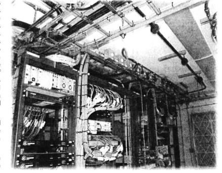
Grounding conductors of all sizes shall maintain a minimum bending radius of 203 mm (8 in.). The angle of any bend shall be not less than 90 degrees.
