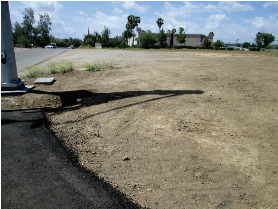
Photo 2: Eastern site boundary along Penfield Lane. Facing south.
