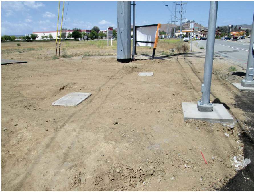
Photo 1: Northern site boundary along Benton Street. Facing west.
