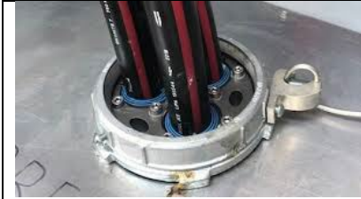
Figure 5.14 Example of optical fiber underground-to-building transition
