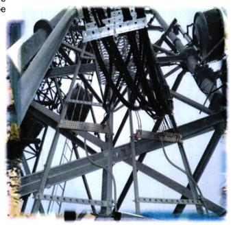
and the jumper cable going to the equipment. The coax protector shall be connected to the ground bus at this point. A SPD shall be used for single station installations and an IS-PT50HN-MA or similar shall be used for installations with combiners.
