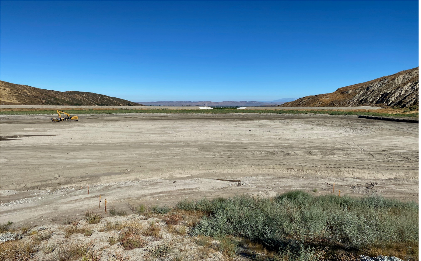
Bautista Creek Sediment Removal
