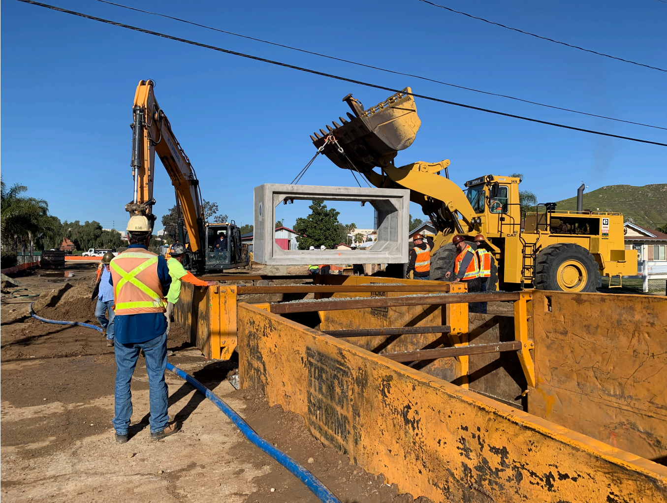
North Norco Channel Line NB, Stg 3
