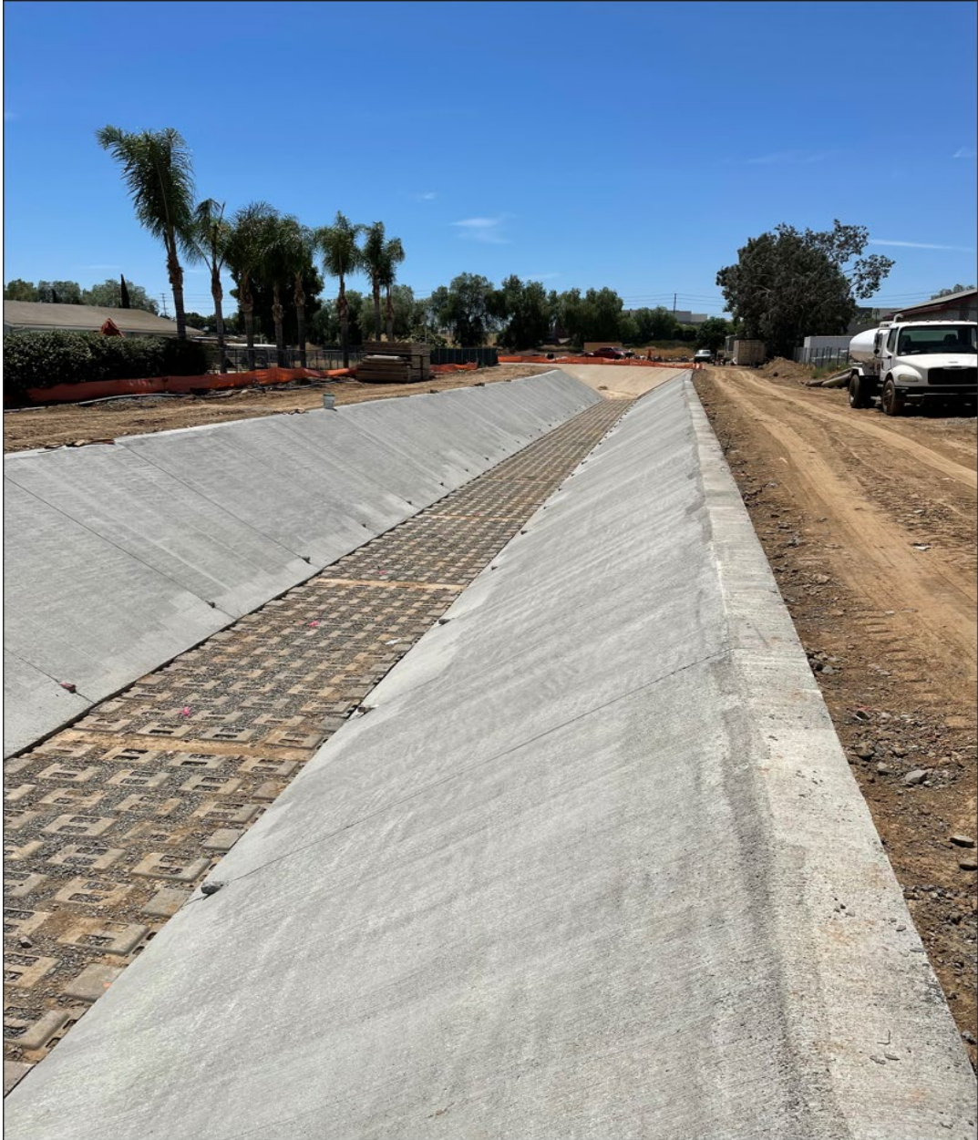
North Norco Channel Line NB, Stg 3
