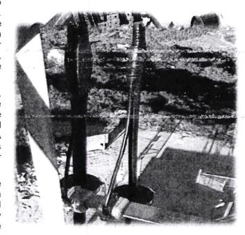
The antenna feed line point of connection to a vertical antenna (Stationmaster type) shall be sealed with electrical tape. A minimum of three wraps shall be utilized. All other types of antennas, with exposed connectors, shall be sealed with Andrew Type 34283 Connector Burial Kit. This shall consist of one wrap of electrical tape, one wrap of Type 34283 Connector Burial Kit and three additional wraps of electrical tape. All wraps shall be properly cut and sealed.
