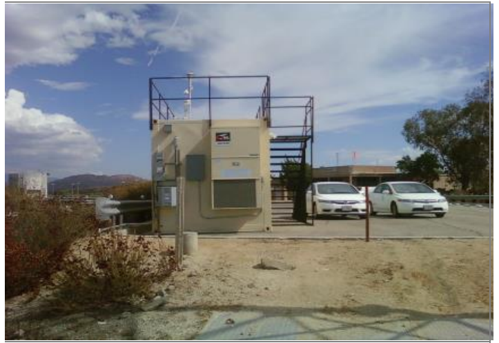
Looking from the probe to the East.
