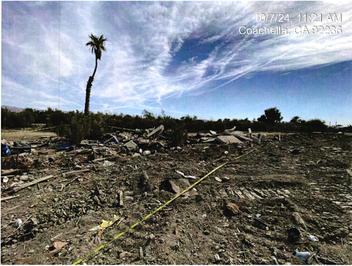
Debris field with positive Asbestos, southeast viewpoint of northeast area of Section G.
