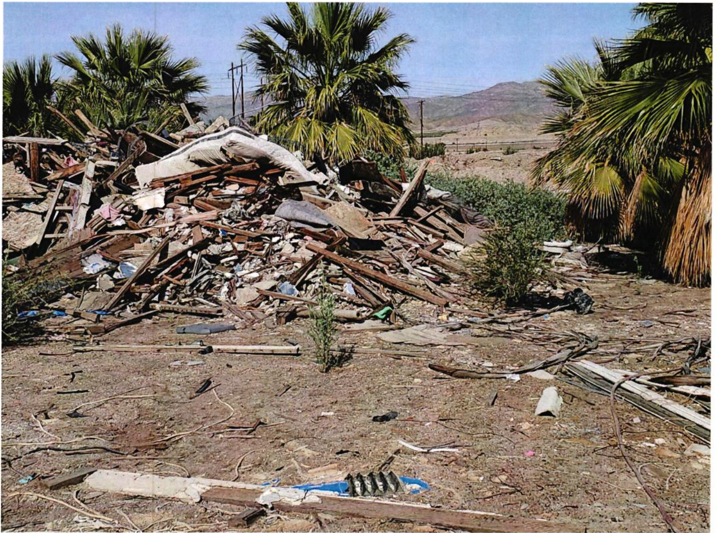
Photograph 16– illustrates Zone E, looking north.
