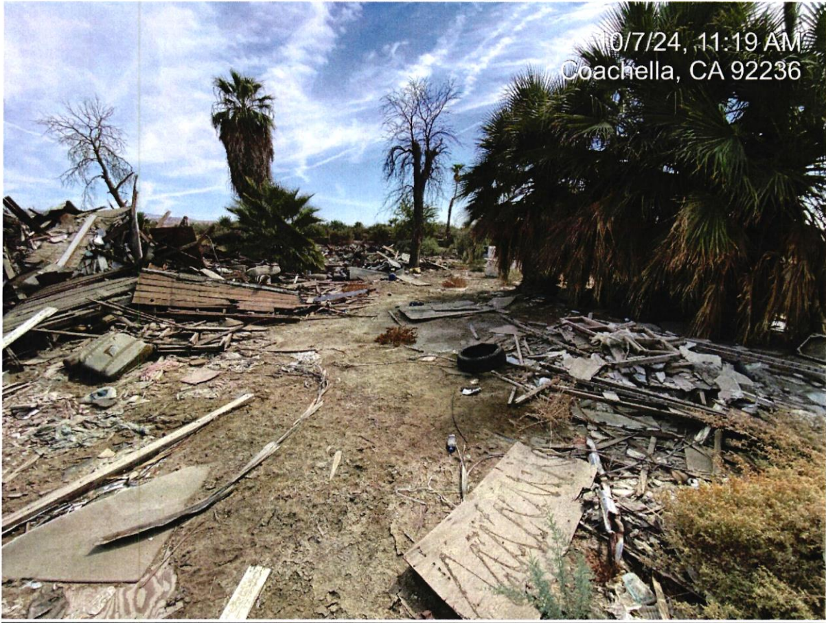
Debris field with positive Asbestos, east viewpoint of southside area of Section F.
