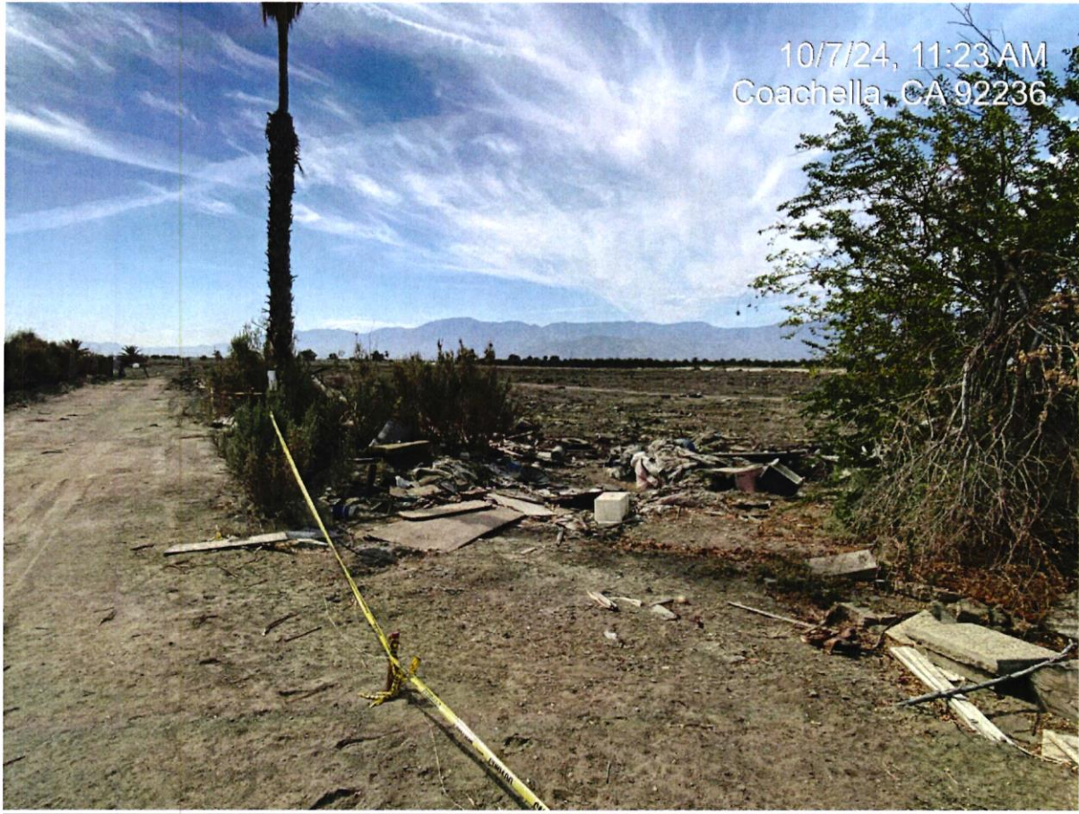
Debris field with positive Asbestos, south viewpoint of northeast corner of Section G.
