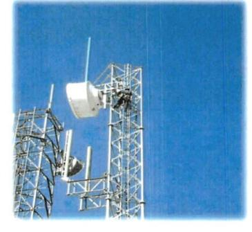
All antenna feed line runs to be installed on towers shall follow the appropriate antenna feed line ladder support. This is dependent upon which side of the tower the antenna is to be mounted. Accordingly, inside and outside positions on the cable ladder shall be evenly utilized when making antenna feed line installations. All antenna feed line runs shall be secured to the antenna feed line ladder and ice bridge.
