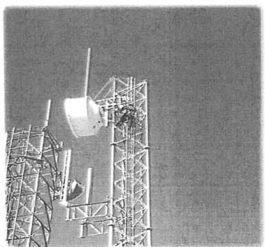
All antenna feed line runs shall be secured to the existing Unistrut brackets with HOT-DIP GALVANIZED Unistrut clamps and STAINLESS STEEL hardware.
