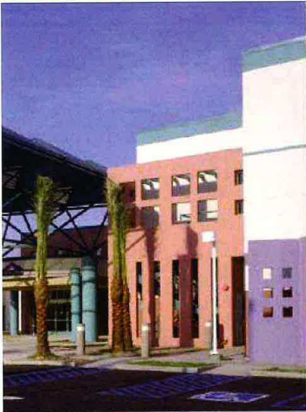
Exterior stair is hidden behind a screen wall of the primary building
