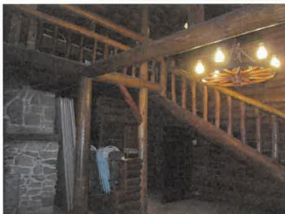
Photo 14- Another interior view with the fireplace on the left. The column under the cross beam was added later.
