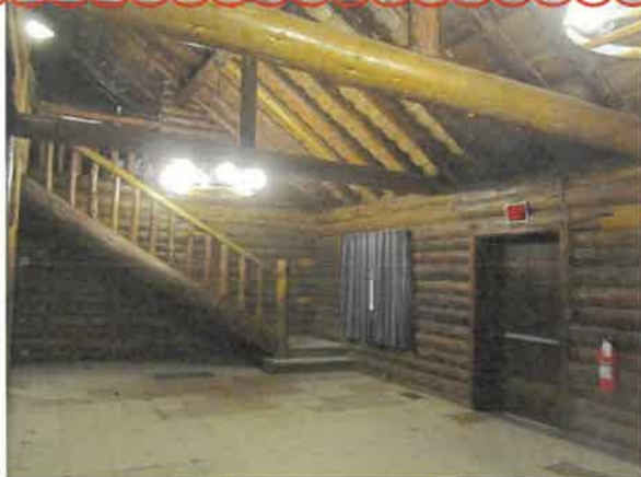
Photo 13- Interior view of main room. This shows the rafters, purlin, posts, and cross beams as well as the wall construction.
