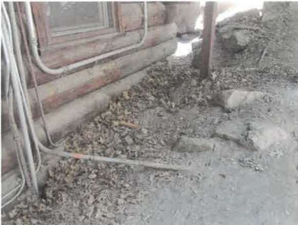
Photo 6 - East wall showing dirt and debris piled around the building.
