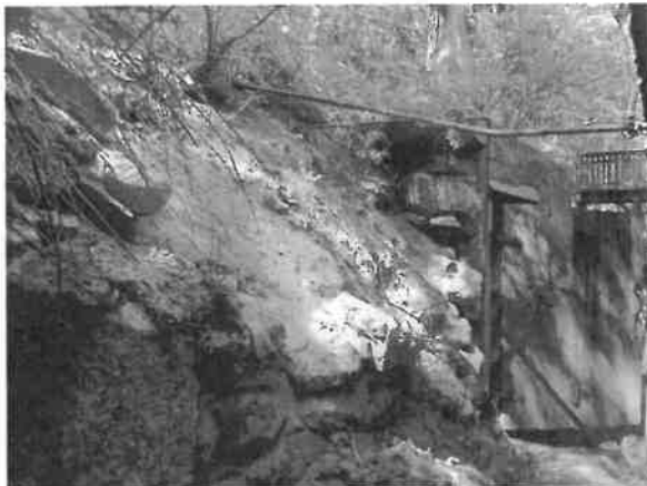
Photo 4 - North side of building. Water draining from the trail has caused rocks to fall into yard space and continues to have sand and gravel sliding down.
